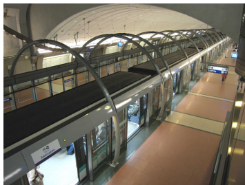
Operating System of Driverless Subway (Paris, Line 14)
